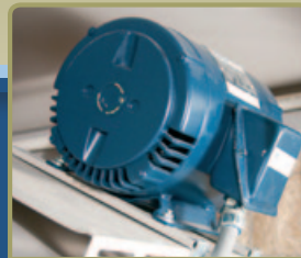
Installation of e.p.a.c.t. motor
