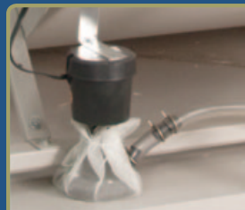
Installation of 115V. Pump
