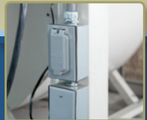
Provision & Installation of 115 V. Receptacles
