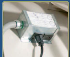
Installation of pump J-Box
