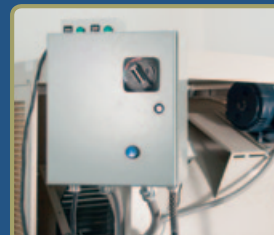
Installation of Weather proof NEMA 3R Box
